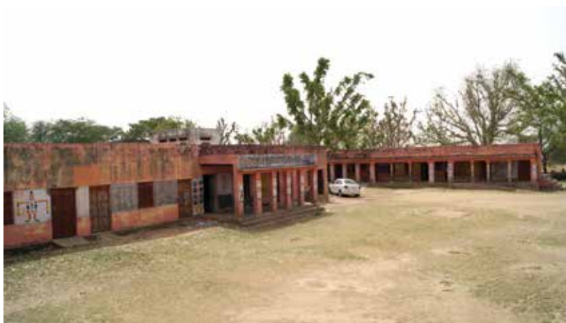
School before renovation
