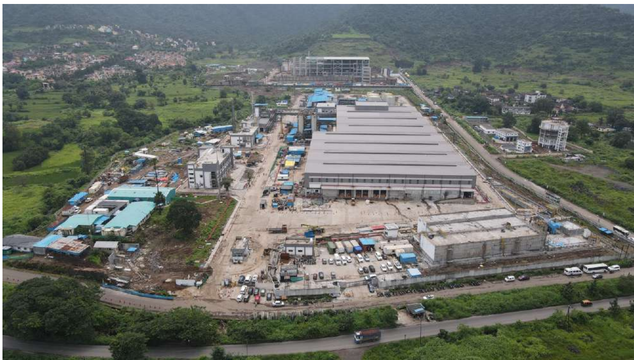
ExxonMobil's upcoming lubricant plant in Maharashtra
