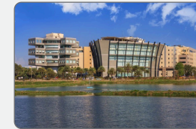
Bagmane Tech Park, Mahadevpura
