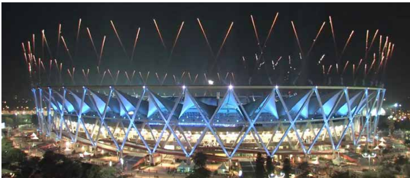
2010 Commonwealth Games: Architectural and Engineering Services for Jawahar Lal Nehru Stadium, Delhi
