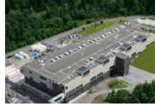
South Hill Data Centre
